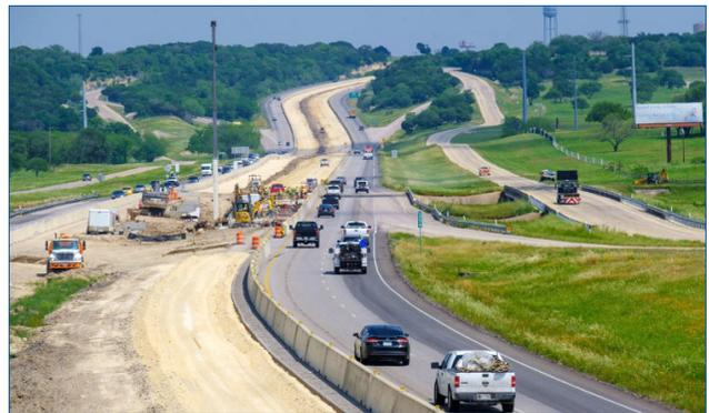
This photo shows road base construction for new lanes and work on widening the Nolan Creek bridge, 7 miles west of I-35.
